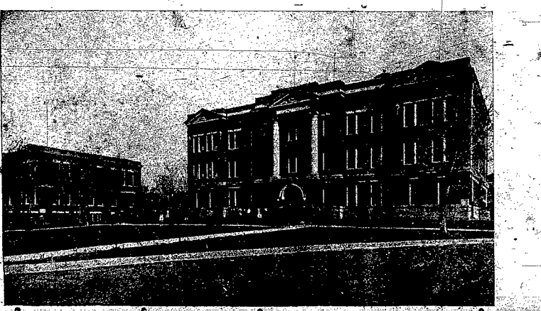
ADMINISTRATION BUILDING WHERE 156 STUDENTS WERE GRADUATED TODAY
